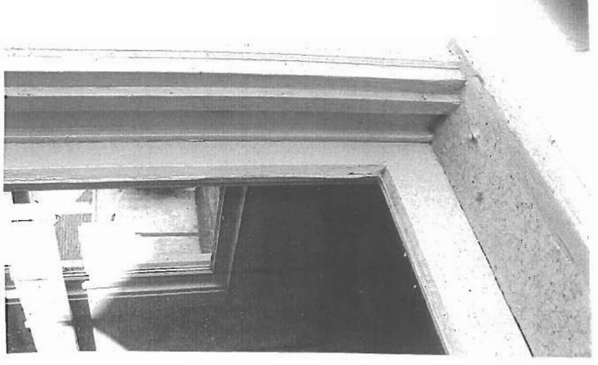
Existing exterior trim →
